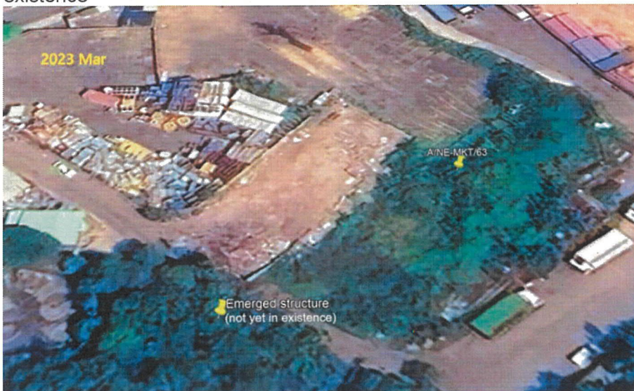
Figure 1. Aerial view of application site taken in 2023 when the structure was not yet in existence
