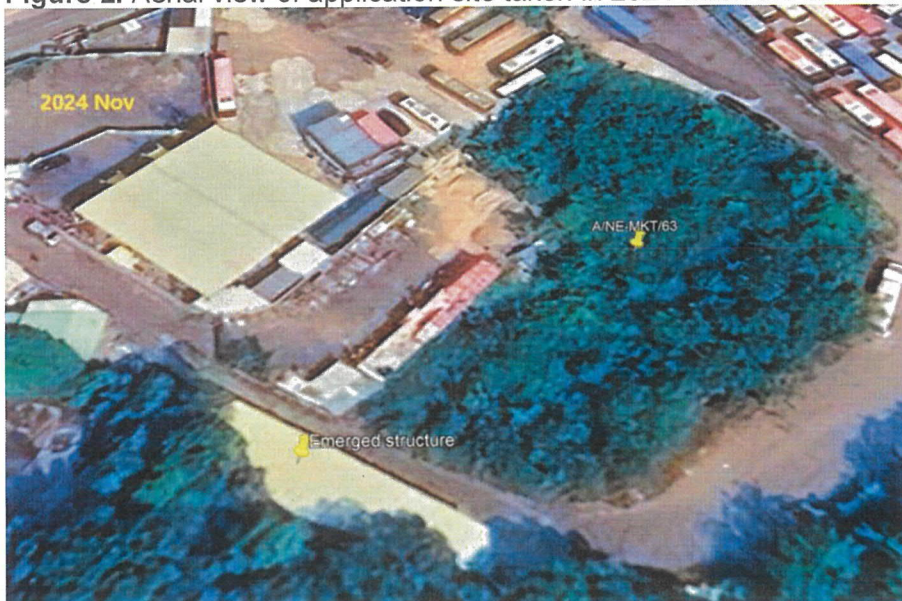
Figure 2. Aerial view of application site taken in 2024 when the structure was in place
